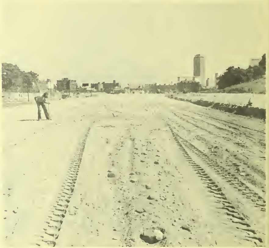
Southwest Corridor Right-of-way looking towards downtown Boston.
